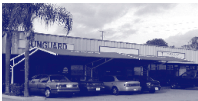
Sunguard Shade Structures Sarasota, FL
