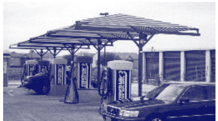
Automation Car Wash Houston, TX
