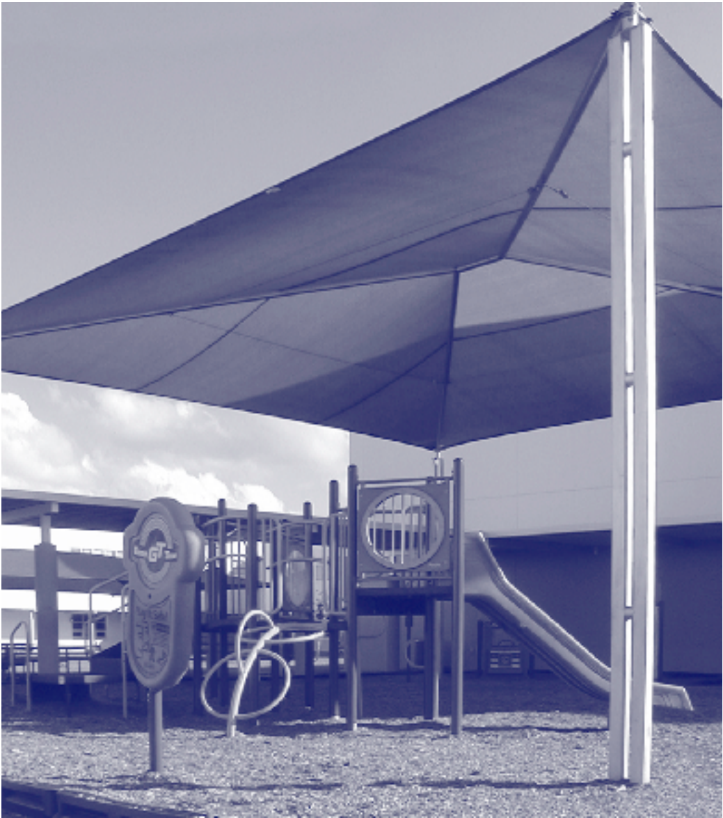
Tuttle Elementary School Sarasota, FL
