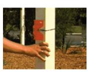
• Before setting the footings in concrete, check all column heights for correct level above and below grade.
