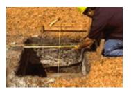
Review footing layout in back of guide. Measure columns for centerline & diagonal. These need to correspond with footing layout details.
