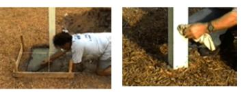
• Clean concrete splatters & residue from the columns & footings.
